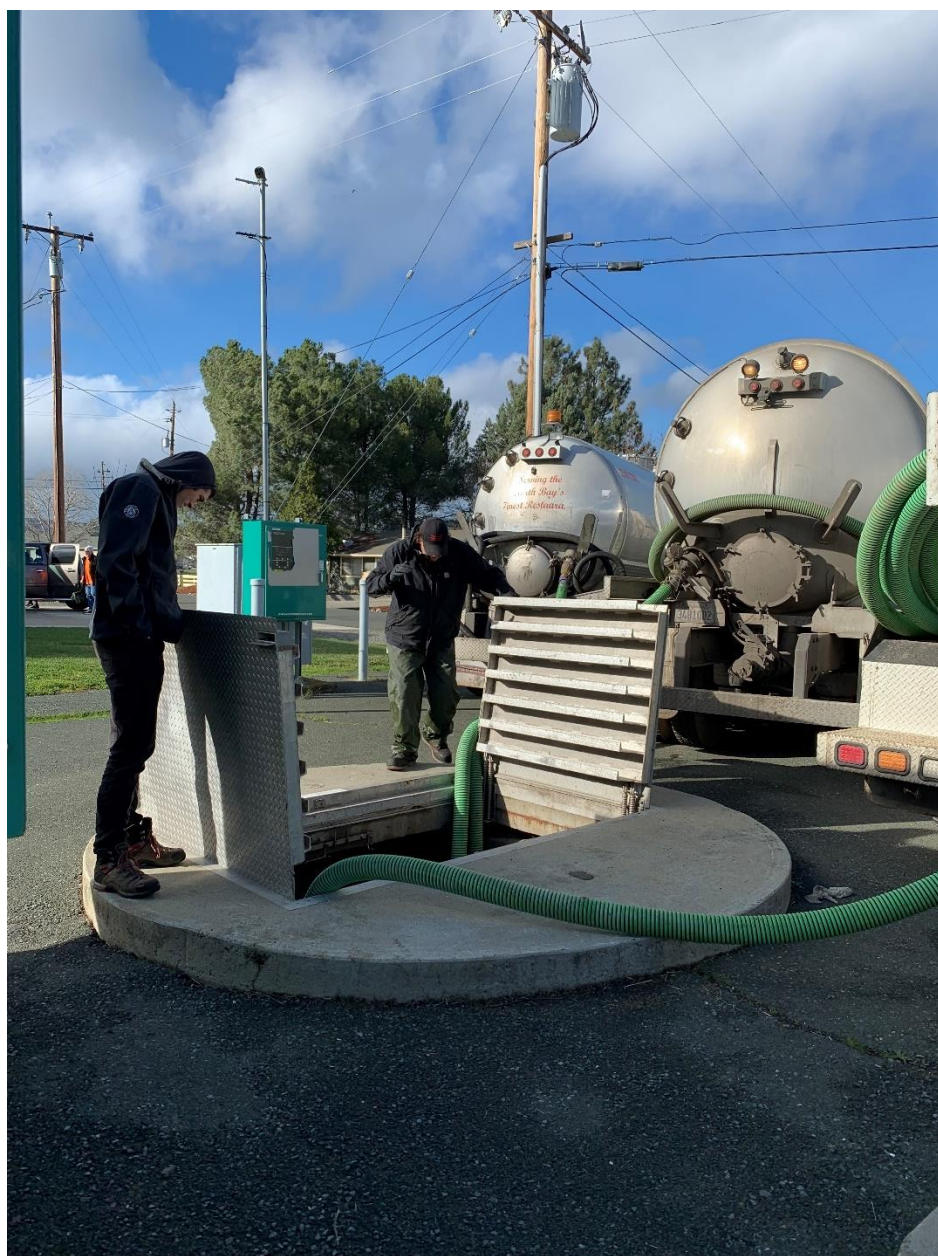
Figure 4-56 HVLCSD – Pumping and Hauling Operations
