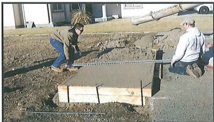
Generator concrete pad being poured.
