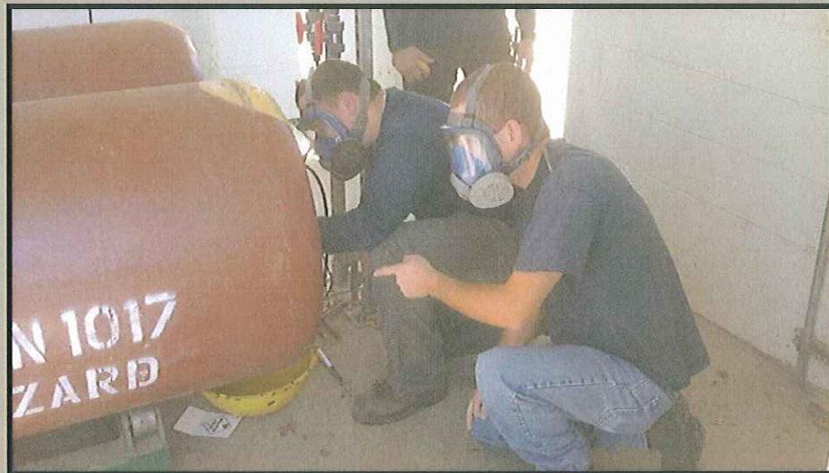
Change out of vacuum hose on 1 ton cylinder chlorine tanks.
