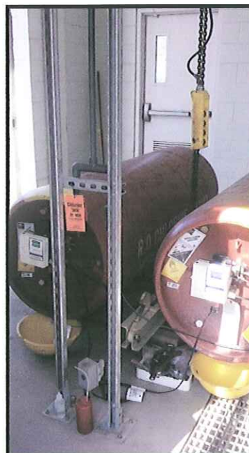
Rack modification in chlorine room.
