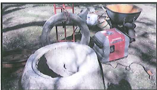
Manhole raised and sealed near Big Beach.
