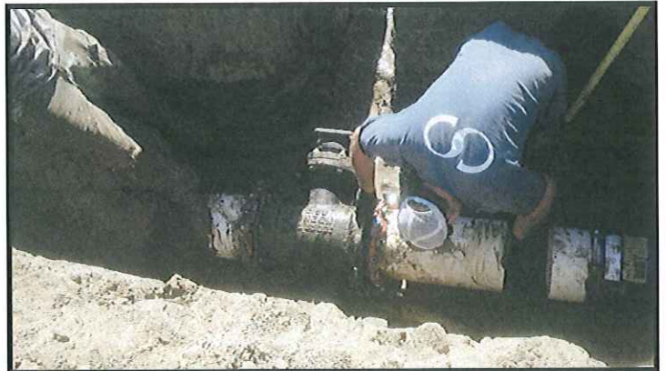
Well #2 tie in.
