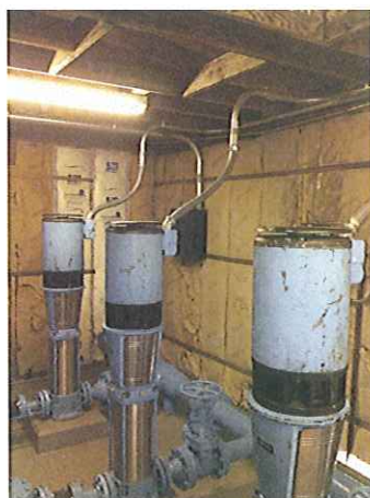
Unit 9 building before work was performed.
