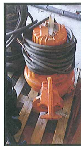
Spare lift station pump for the plant.
