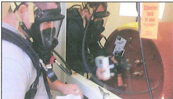
Chlorine cylinder change-out exercise using respirators and proper equipment.
