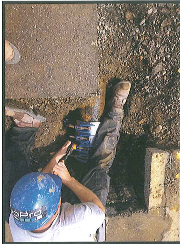
Redbud mainline leak repaired with new saddle on water main.
