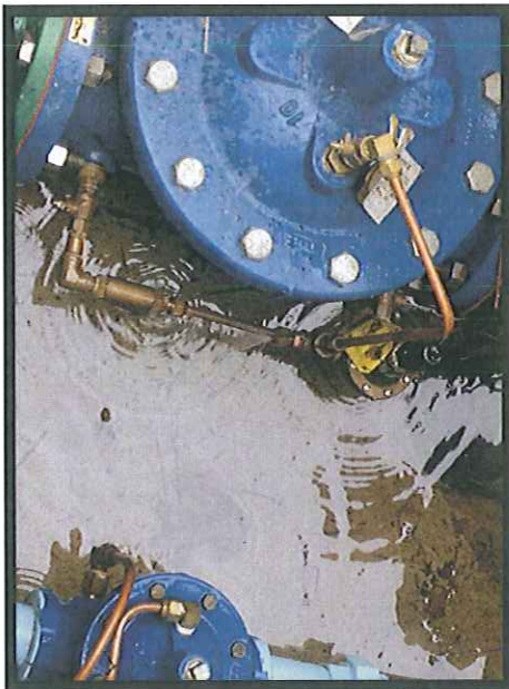
Spruce Grove/Knollview PRV repair.
